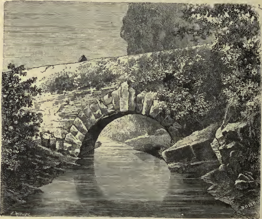
Roman Bridge over the Ostian Road.
